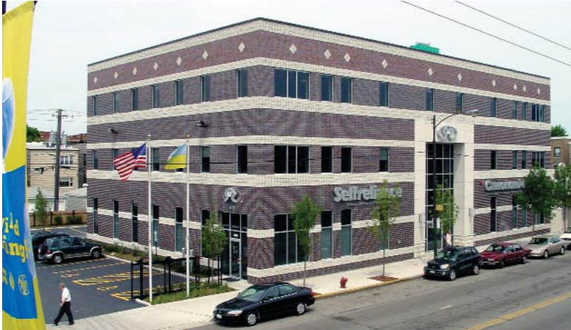
The new Home Office was built on the site of the credit union's former one-story rental property and parking lot at 2332 W. Chicago Avenue. It stands on the north side of Chicago Avenue, across from the former main office.
